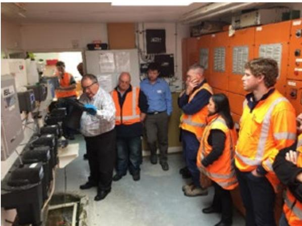
After lunch everyone made their way to the nearby Balclutha Water Treatment Plant which has a UV process. Attendees were split into 2 groups, one doing actual UVT testing of various samples and turbidity unit calibration, the other doing UV sensor verification. When finished the groups swapped. This practical hands-on session was much appreciated by everyone and perfectly augmented all the theory presented in the morning.
